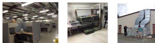
Fig. 4. Test Site I at Joint Base Lewis-McChord
